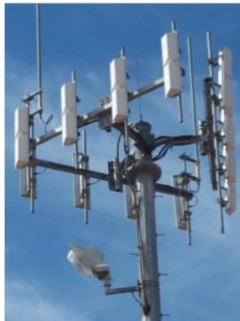
Triangular array of dipoles used as a sectoral antenna in base-station antenna for mobile communication.
