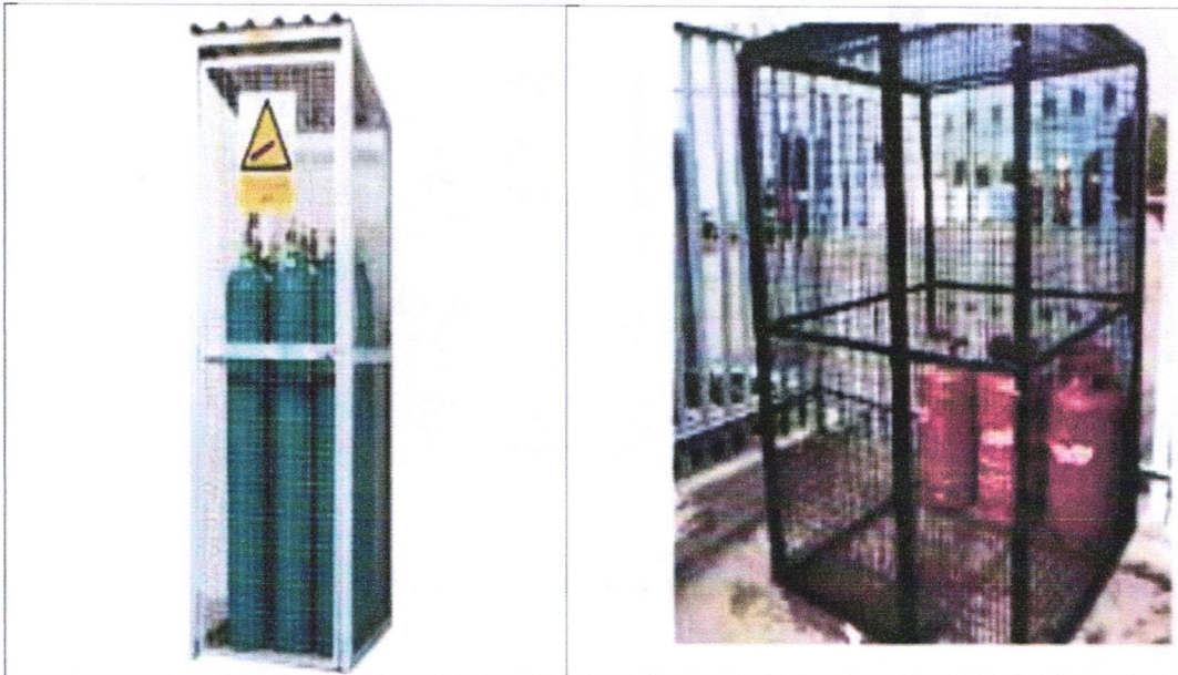
Figure-38 Safe storage of gas cylinders.
